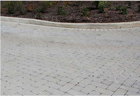
Permeable paver system
