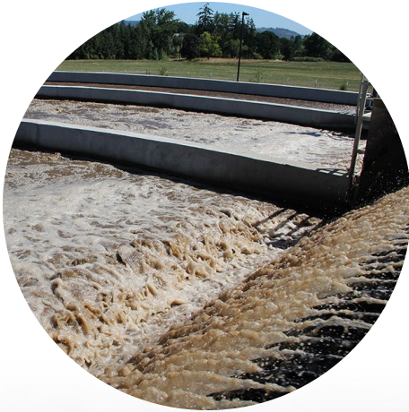
Oxidation ditch aeration basin with three zones.
