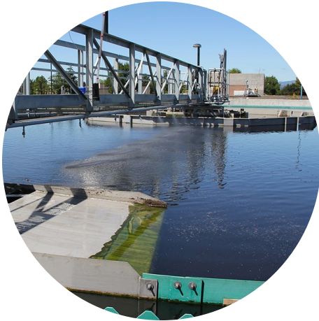
New stainless steel scum beach for new secondary clarifier.
